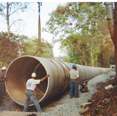
Top: The lightweight HOBAS fiberglass pipe sections were carried to the point of installation and assembled using the single excavator visible in the background. Bottom Left: Field service crew assist the installation contractor. Bottom Right: The high strength and corrosion resistant FRP pipe has many advantages in Penstocks.
