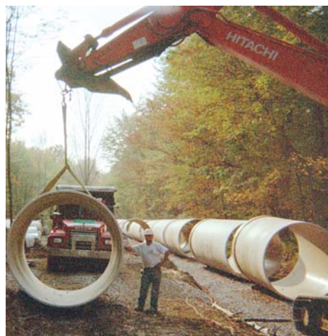
Top: The lightweight HOBAS fiberglass pipe sections were carried to the point of installation and assembled using the single excavator visible in the background. Bottom Left: Field service crew assist the installation contractor. Bottom Right: The high strength and corrosion resistant FRP pipe has many advantages in Penstocks.
