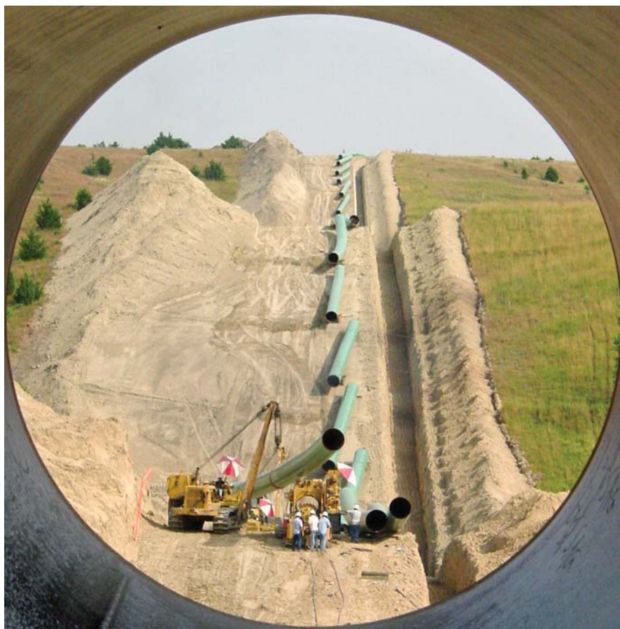
REX West Construction photo by Butch Stovall
