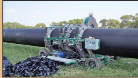
McElroy 1648 MegaMc fusion machine operated by Gajeske Inc.
