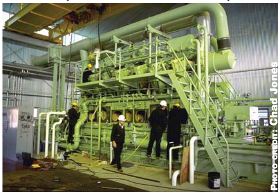
Questar personnel working on a reciprocating transmission and storage compressor.
