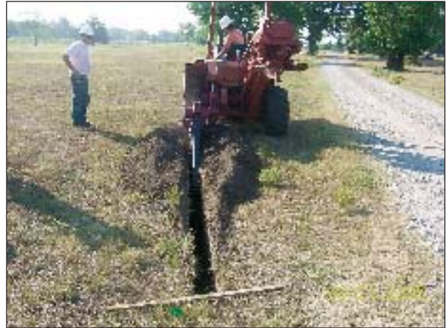
Installation of MATCOR Linear SPL™-Anode at a Houston site
